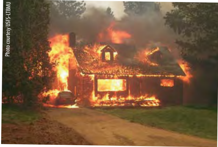
This house was ignited by burning embers landing on vulnerable spots. Notice the adjacent forest is not burning.
